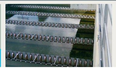
FLOCOPAC®.L by H+E for precipitation and flocculation in industrial wastewater treatment
