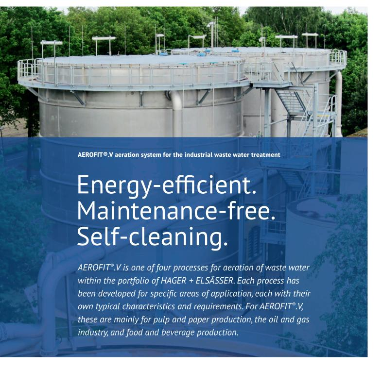
AEROFIT®.V is a medium-size bubble aeration system. It is characterised by particularly high oxygen transfer efficiency, long service life and a wide control range, whilst maintaining a consistently high level of efficiency. Thus, AEROFIT®.V offers decisive advantages over membrane aeration. AEROFIT®.V can be used for surface aeration as well as in spiral flow, whilst at the same time
