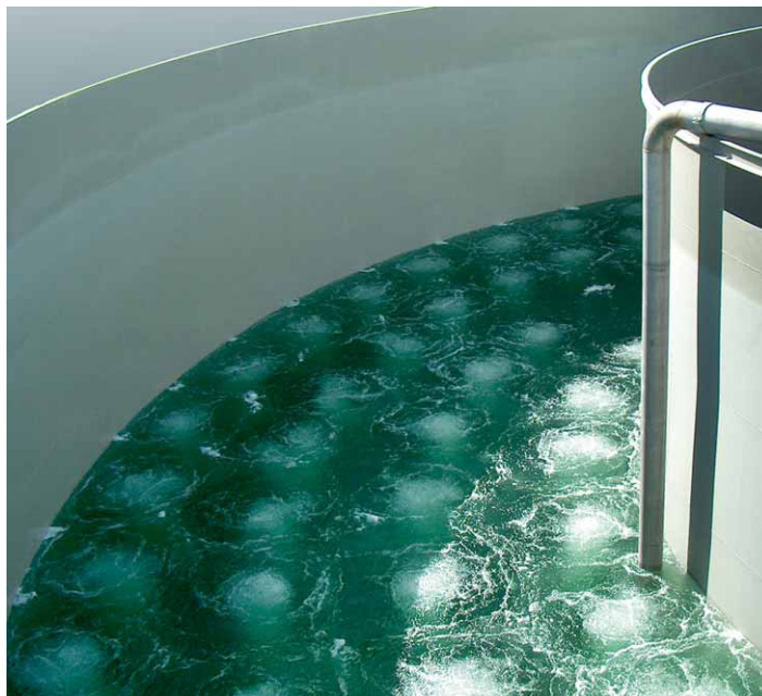
Nitrification stage of BIOFIT®.N with AEROFIT®.D aeration system in a test run
